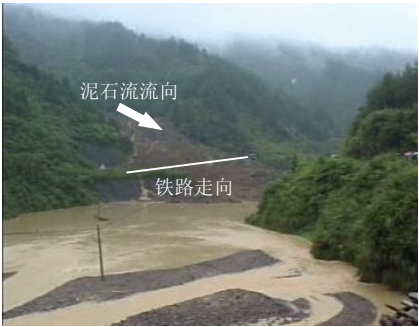
图 4 卓福泥石流暴发后地貌 Fig.4 The geomorphology after Zhuofu debris flow
